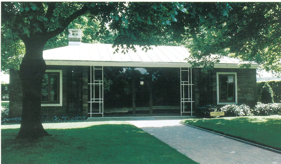
Visitors' and Office Building
